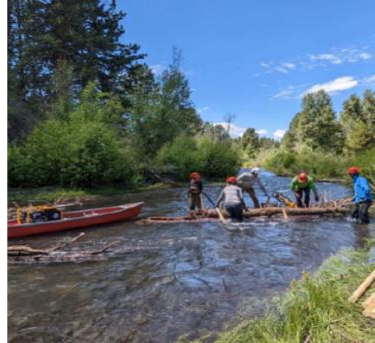
Post assisted log structure, Eastern Oregon
