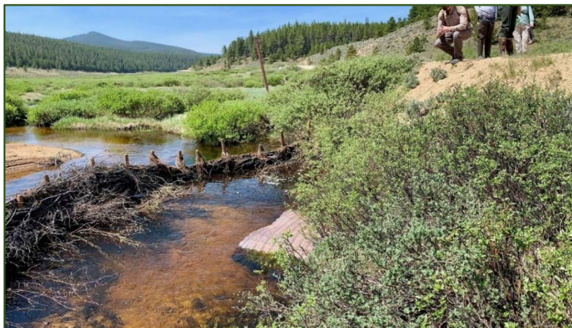
Photo by Jackie Corday, a “starter dam” installed to protect a road culvert.
