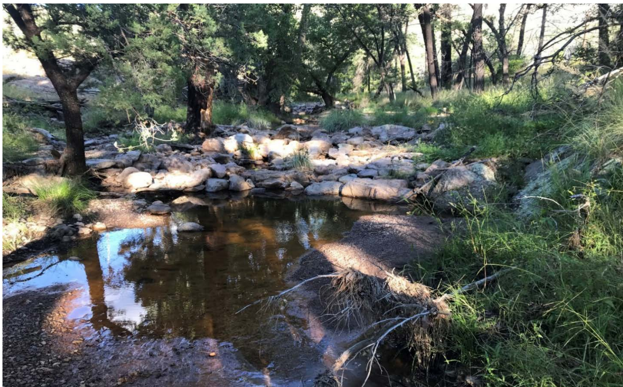
Photo of an example of a rock detention structure on an Arizona creek provided by Dr. Laura Norman from the June 2022 video Re-greening a Dryland Watershed | U.S. Geological Survey (usgs.gov) .
