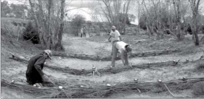
Workshop volunteers build a wicker weir on Largo Creek, Williams Ranch, Quemado, NM. August 2024. Photo by Tamara Gadzia. Slide from the presentation: An Introduction to Induced Meandering: A Method for Restoring Stability to Incised Stream Channels, Zeedyk, Earth Works Institute and Quivira Coalition, (2009).
