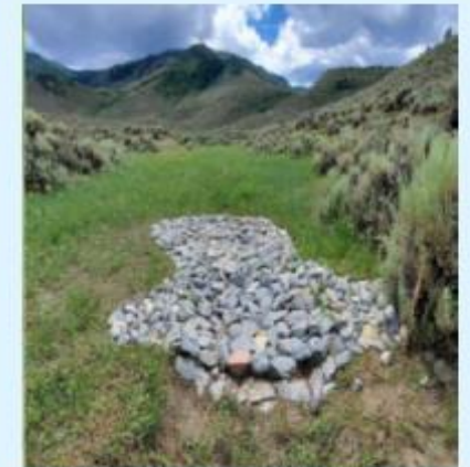
Project photos from Shawn Conner, BioLogic
