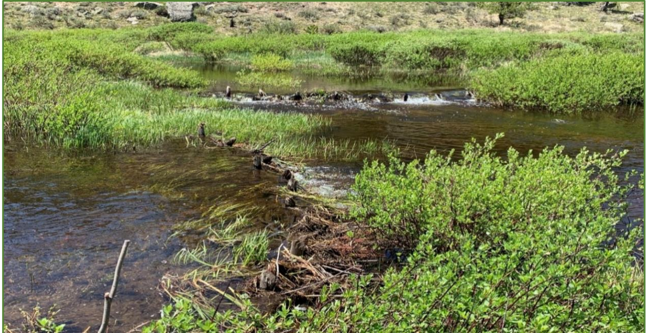
BDAs installed in Sept. 2021 on Trail Creek in the Upper Gunnison Basin. This is a great example of a project carefully designed to avoid conflicts with its location high in the headwaters above reservoirs and diversions, and notice how short and porous the BDAs have been designed. Photo taken in June 2022 by Jackie Corday
